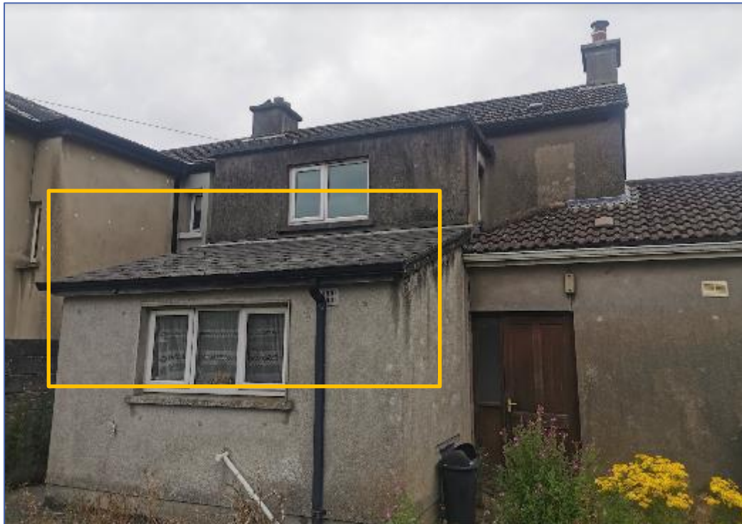
Asbestos Roof Slates
