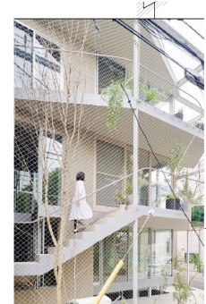
4 STAIRCASE ENCLOSED IN MESH SCREENING
