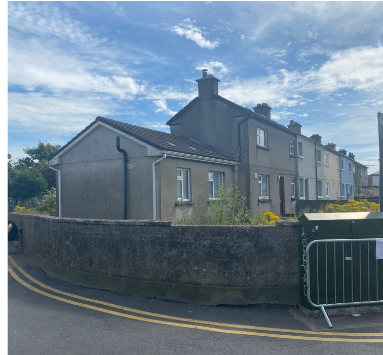
View of side extension (to be demolished)
