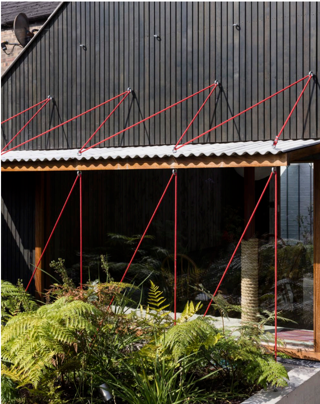
Reuben St, Dublin by TAKA Architects
