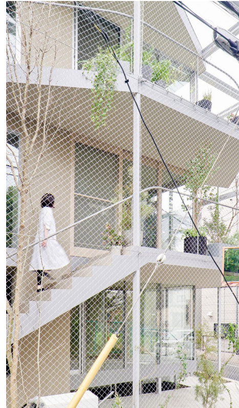
Staircase enclosed in mesh screening
