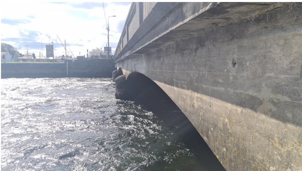
Plate 3-2: Side of bridge lacks crevices suitable for roosting bats.
