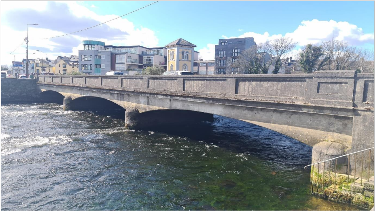
Plate 3-1: Wolfe Tone Bridge
