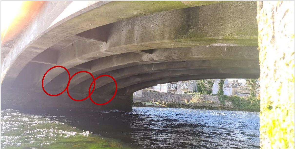
Plate 3-9: Areas of bridge where bat droppings were found.
