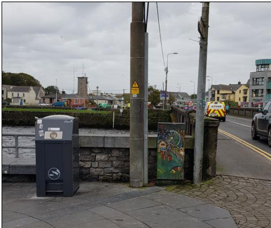
Photograph 8 - Eastern Abutment (Southern Side)
