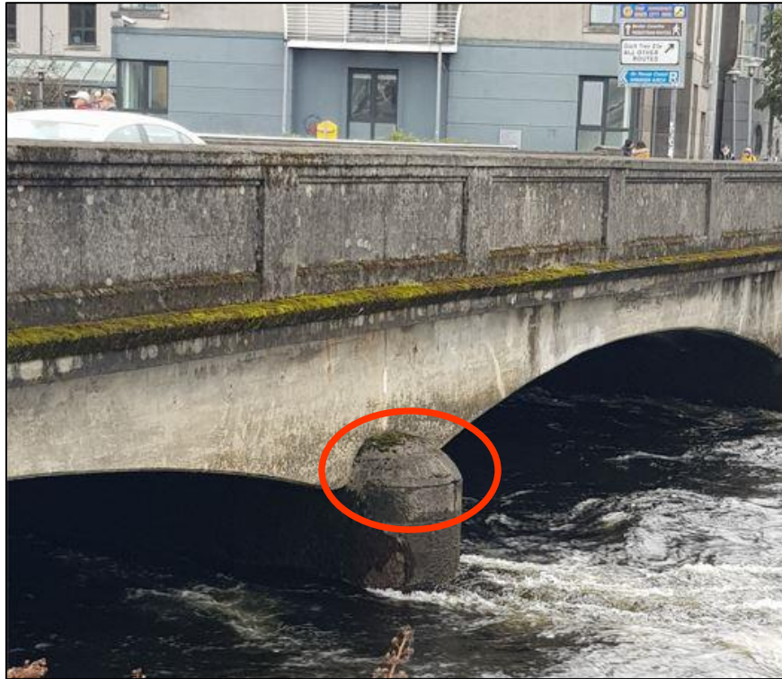
Photograph 1 - Top Stone of Existing Piers and Abutments to be Removed
