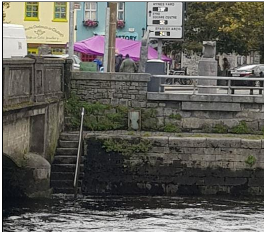
Photograph 6 - Eastern Abutment (Southern Side)
