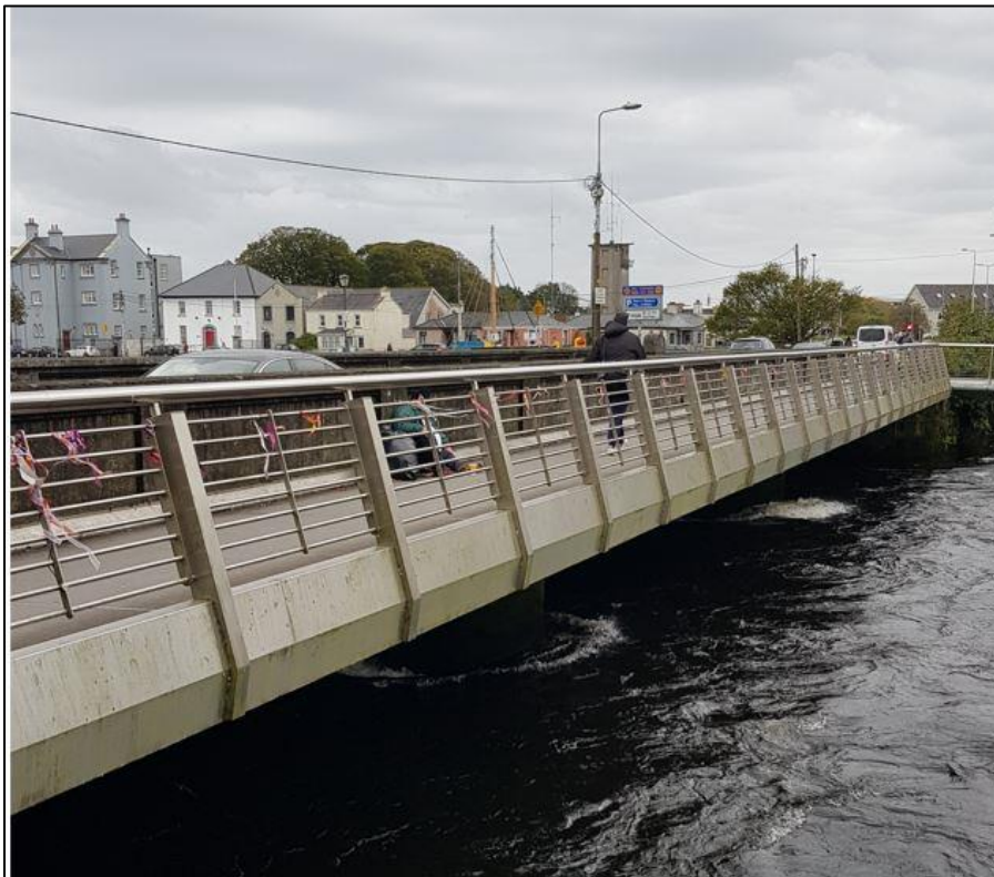
Photograph 4 - Existing North Side of Bridge (Upstream)
