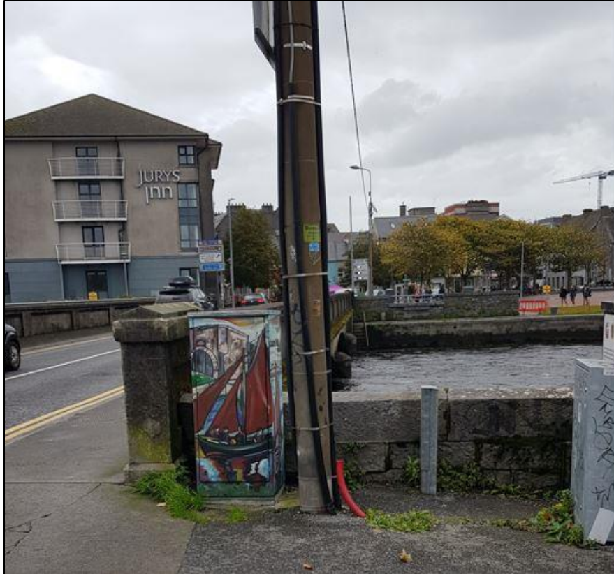
Photograph 7 - Western Abutment (Southern Side)
