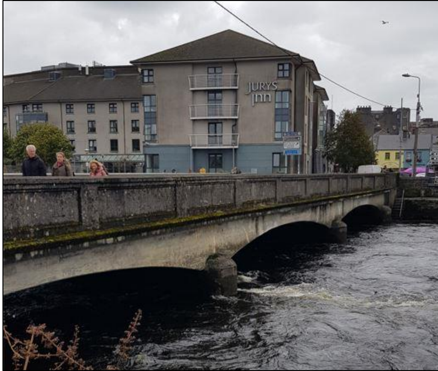
Photograph 3 - Existing South Side of Bridge (Downstream)
