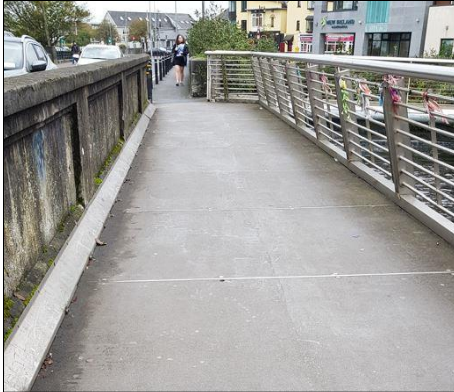
Photograph 5 - View of the Existing Cantilevered Walkway (facing SW)
