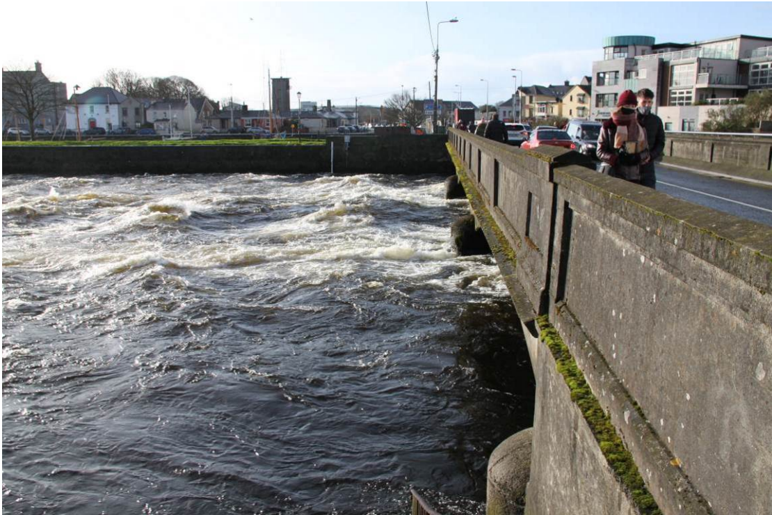
Photo 5 View From East Abutment
