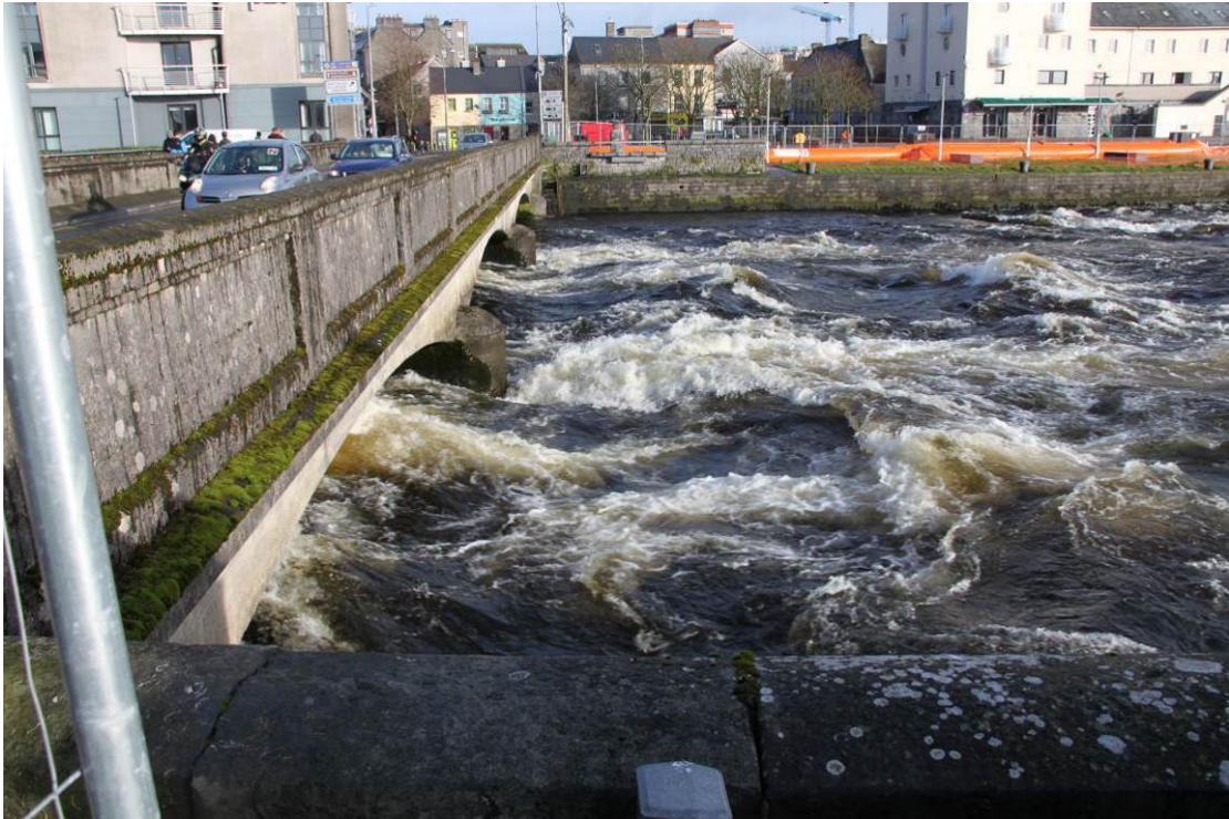
Photo 3 View From West Abutment
