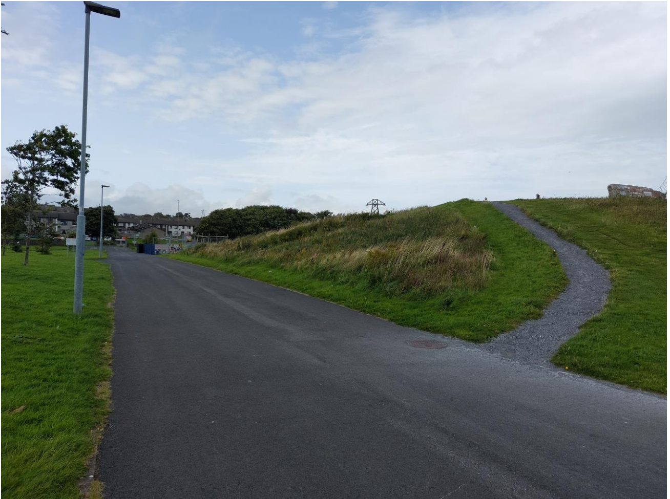
Photo 4 Artificial surfaces and existing lighting along footpath
