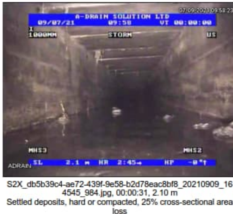
Figure 2 Internal Photo of Culvert - Adrain Solutions CCTV Image
