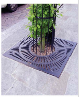
08: Cast iron tree grill.
