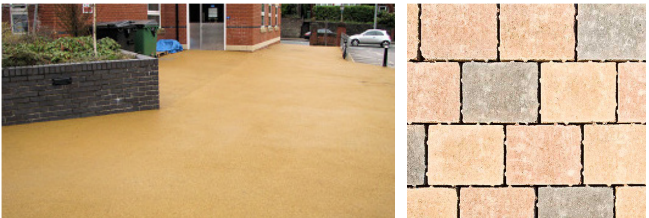
Fig's. 10 & 11 Show Buff coloured SMA and permeable concrete pavers
