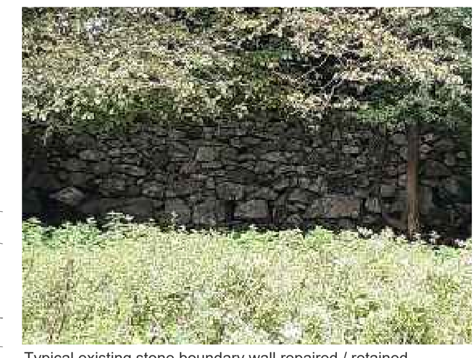
Typical existing stone boundary wall repaired / retained.
