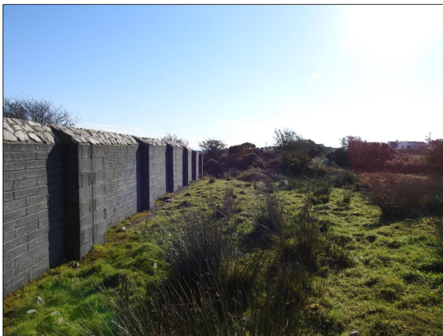
Plate 13 There is a blockwork wall along the northern boundary.
