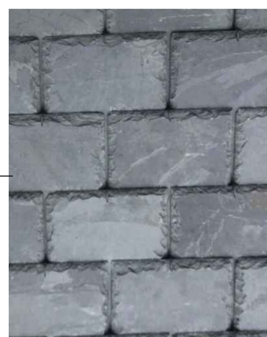
NATURAL SLATE ROOF
