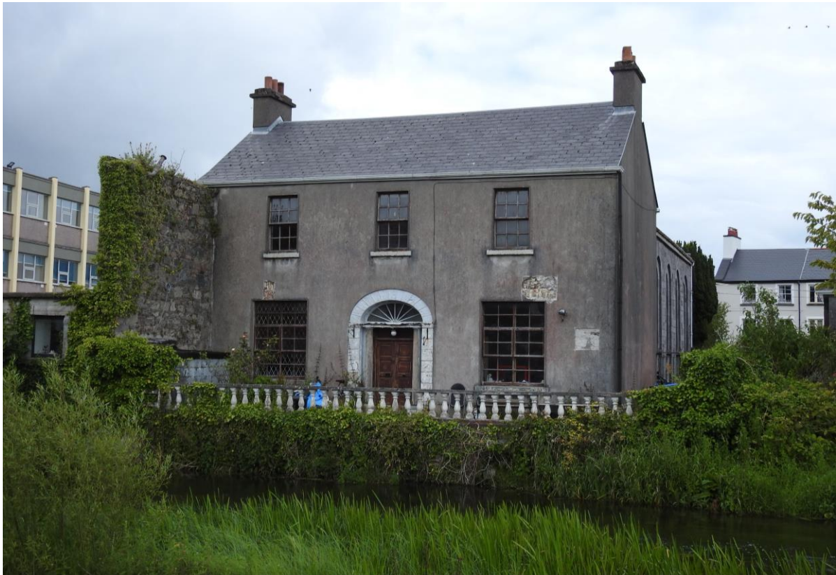
Fig.2: Front or west facing view of Church House, Galway.
