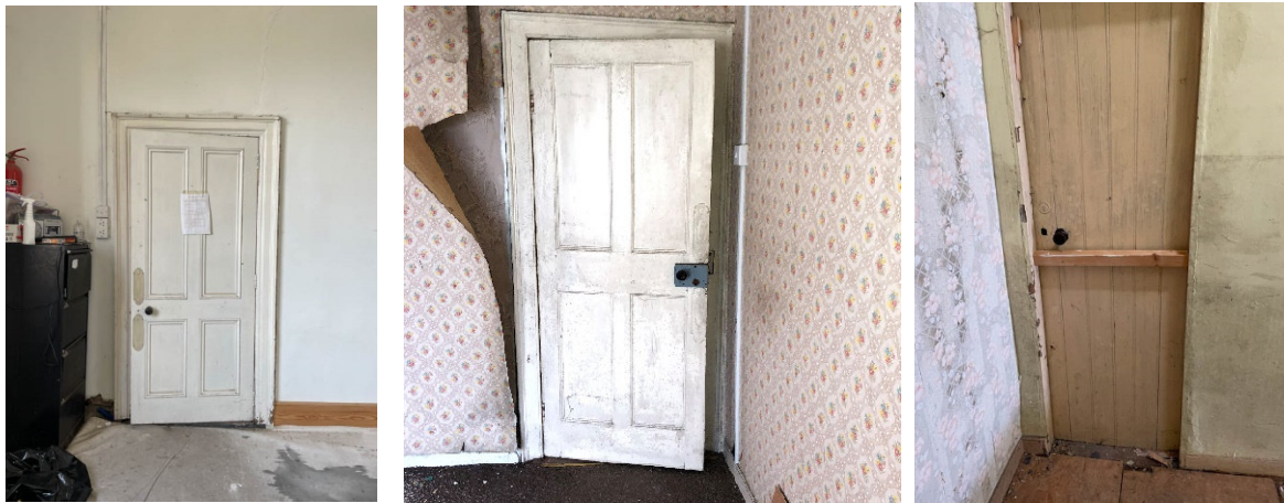
OBFA photos of existing main Manse internal doorways
