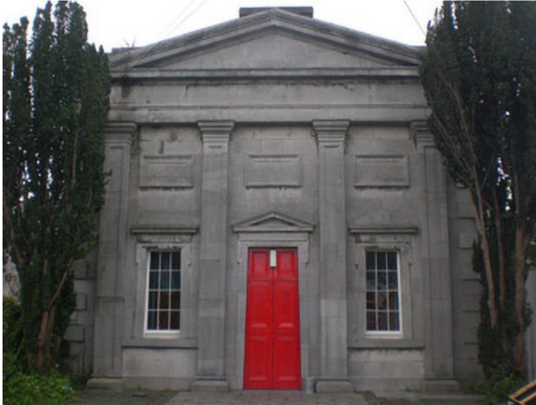
Photo of the front Façade of The Presbyterian Meeting Hall, now Nun's Island theatre from NIAH website. Building designed by James Cusack.
