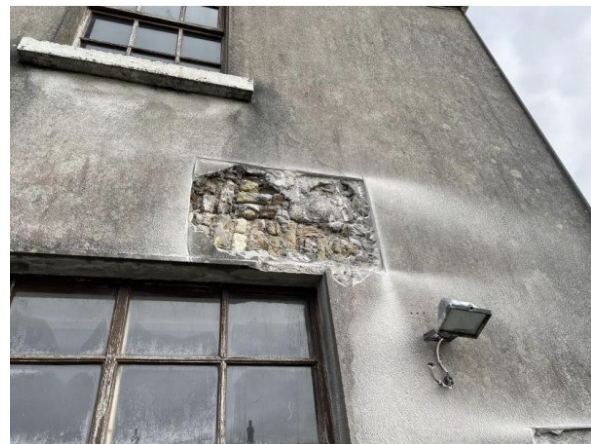
McKennas Photo of External Wall opening -Manse
