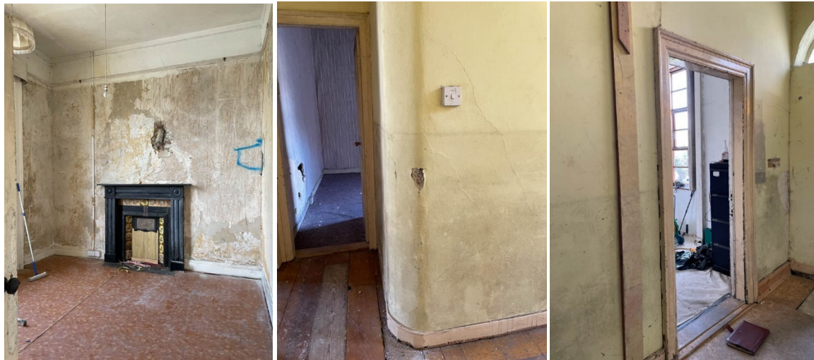
OBFA photos of existing main Manse internal framing
