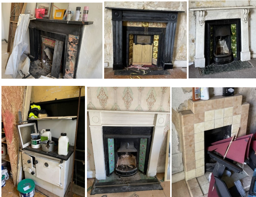
OBFA photos of existing main Manse fireplaces & stove
