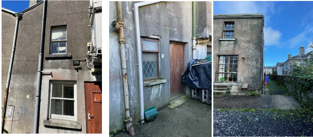
OBFA photos of existing external Manse windows
