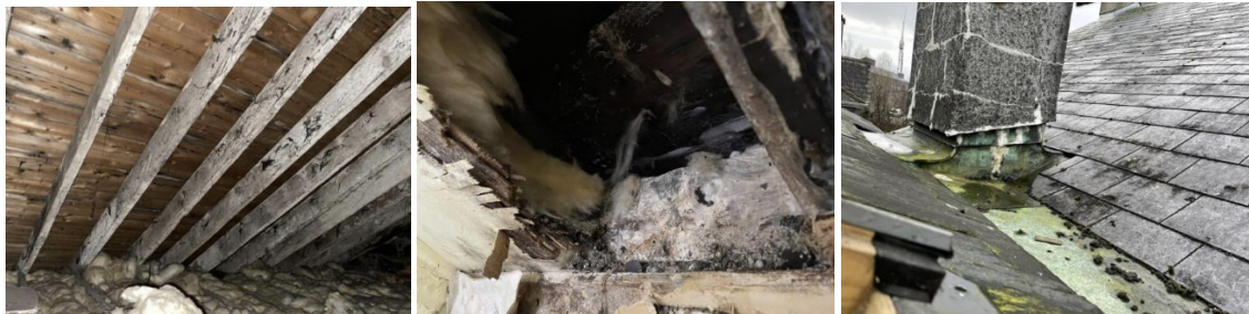
McKennas photos of existing roofs
