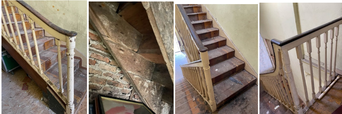
OBFA photos of existing main Manse stairway
