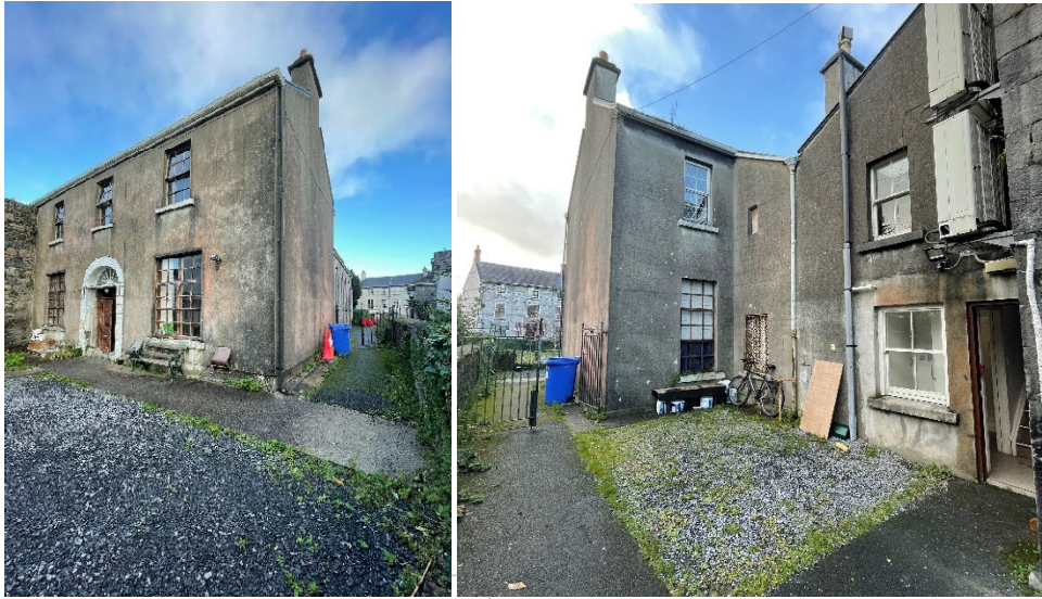
OBFA Photos of existing "Manse" from the riverside and from area to the south of the link
