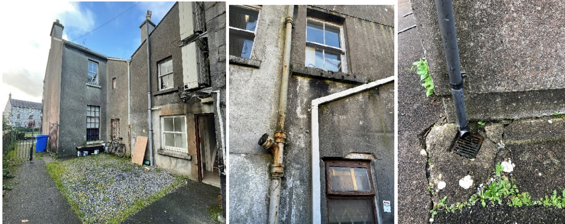
OBFA photos of existing external Manse Chimneys & surface pipework
