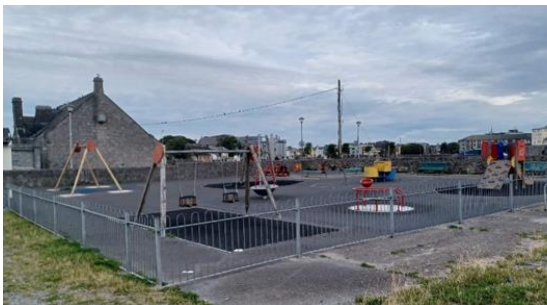
Claddagh Playground - Before
