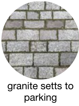
granite setts to parking
