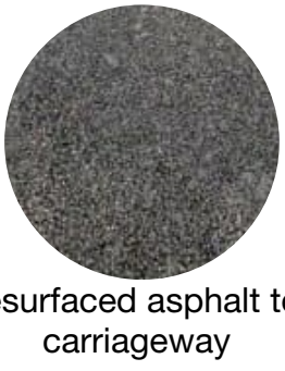
resurfaced asphalt to carriageway
