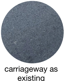
carriageway as existing
