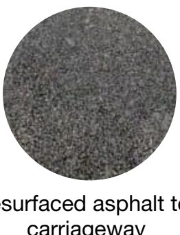
resurfaced asphalt to carriageway
