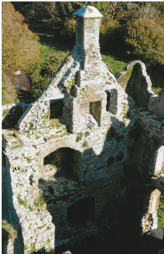
Fig. 85 The interior of the surviving gable of the tower house is attached to the 17 th century Renaissance style façade (on right) and a very thick side wall on the left which could be incorporate tower house fabric as well as the walling of an earlier hall-house type castle.
