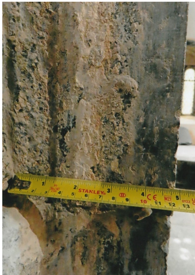
Fig. 68 Layers of lime wash on the moulded side of the canopied wall-tomb.
