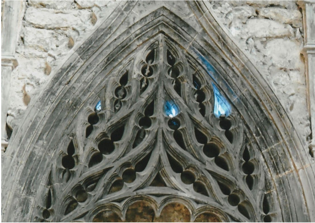
Fig. 67 The tracery of the flamboyant Gothic Style Canopied and Traceried Wall Tomb Lights have been inserted to show the line of a cut stone recess with a chamfered edge occurs behind the upper part of the tomb. It is unclear whether this feature continued on either side as the tomb recess is blocked with stone mortar and a (19th century) tile.
