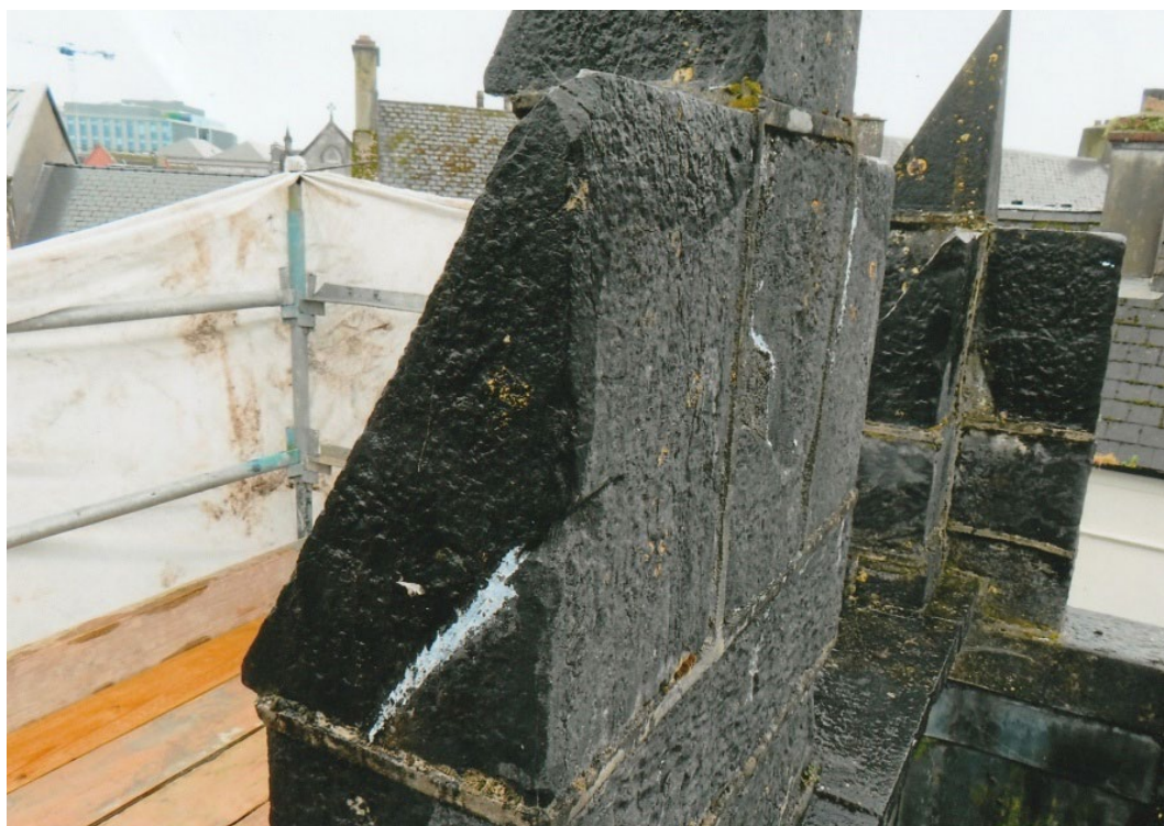
Fig. 8 The crenellations are of several dates and have been re-set. Mastic used to repair breaches in the stone in the 1990's or 2000's was removed and replaced with lime mortar. Photograph: J. Higgins.
