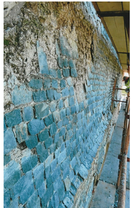
Fig. 75 The schist weather sheeting on Menlo Castle. Ivy growth had dislodged many slates prior to its removal in 2021.
