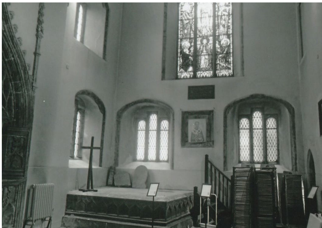
Fig. 39 The Southern Extension to the South Transept at St. Nicholas' Collegiate church before the 2023 conservation work. Work on stripping the plaster internally was carried out in September and early October 2023 and included an area on the east side of the southern end of the Transept extension above the Lynch 'Corner Tomb' which bears the arms of Lynch and Athy and including the area around the two windows on the right of the photograph and around the Flamboyant Canopied and Traceried Lynch Wall-Tomb, part of which is visible on the left side of this image. Photograph: J. Higgins 2022.
