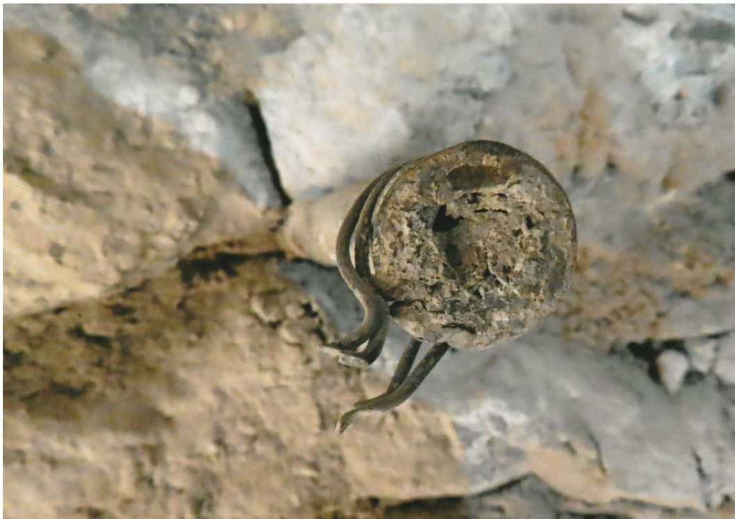
Fig. 59 The wire was threaded through wooden shuttering while the concrete was inserted in the fill of the wall-niche.
