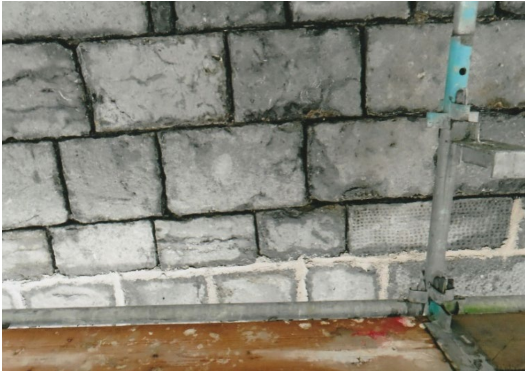
Fig. 30 Stone work on the exterior of the South Transept Extension. Photograph: J. Higgins.
