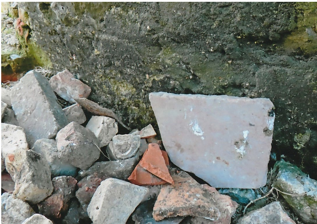
Fig. 104 Paving, roof ridge fragments, slate and brick in advance of cataloguing Menlo Castle 2023. Photograph: J. Higgins.
