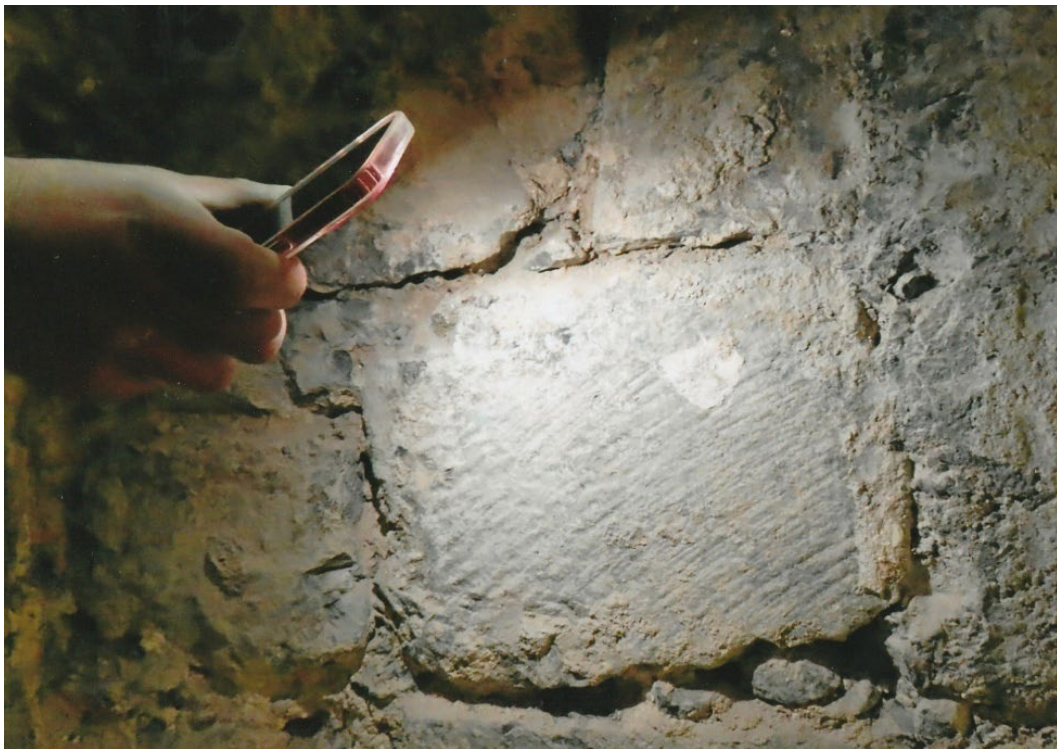
Fig. 10 Ashlar block with diagonal tooling of a type common between the 12th and 14th centuries incorporated in the rectangular projection from the wall. This occurs 297cms above ground level. It and 15th – 16th century worked stone has been reused in the walling supporting the flamboyant Lynch canopied and traceried wall tomb.
