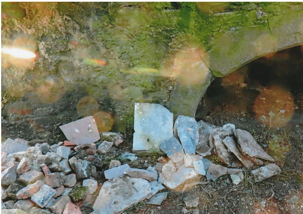
Fig. 101 Reused schist roofing slates, Blue Bangor and Killaloe slate at Menlo Castle. Photograph: J. Higgins.
