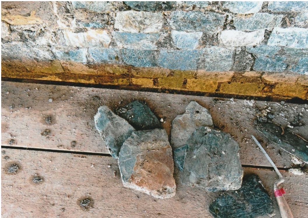
Fig. 91 Detached weather sheeting slates which fell when the ivy was removed are being put back. Note the nail holes in some of the slates. Photograph: J. Higgins.
