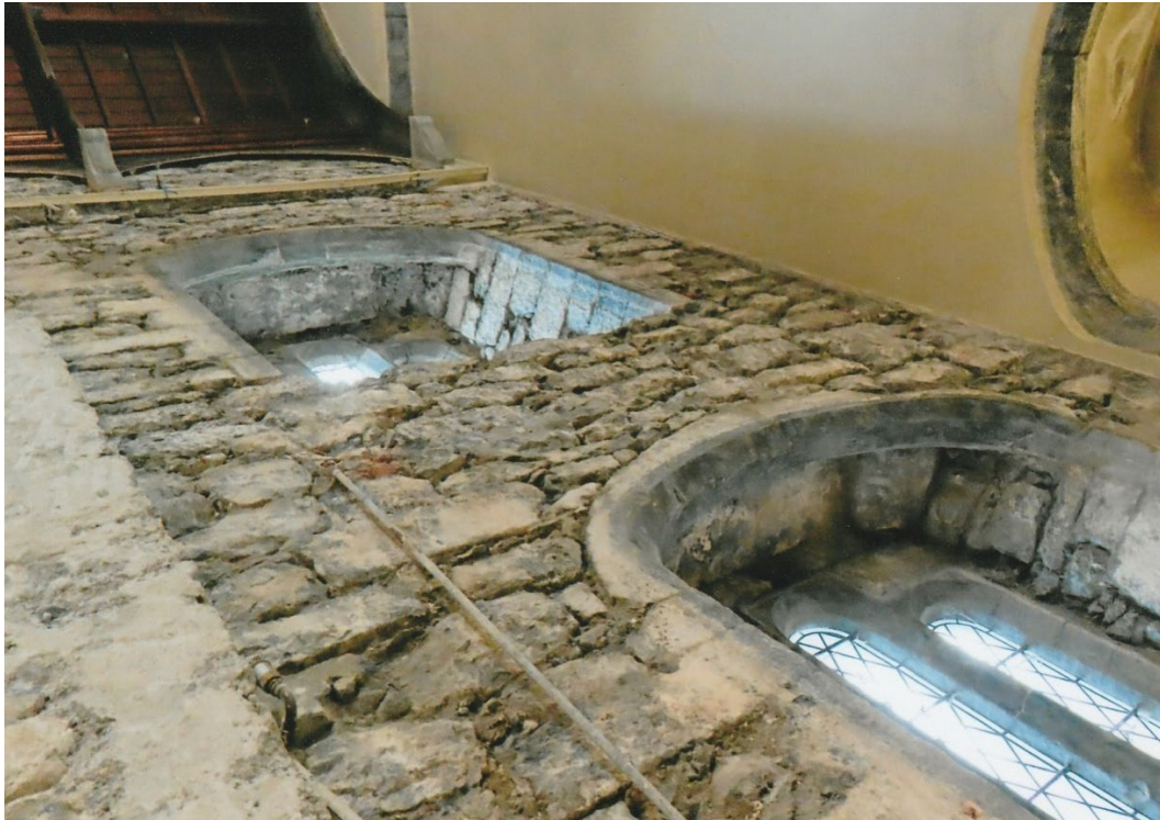
Fig. 54 The windows in the east wall of the South Transept Extension as revealed in October 2023. The lintels were used instead of an arch in the core of the wall. Flat slabs and cantilevered stones and packing including some reused stone was used to support the window heads internally.
