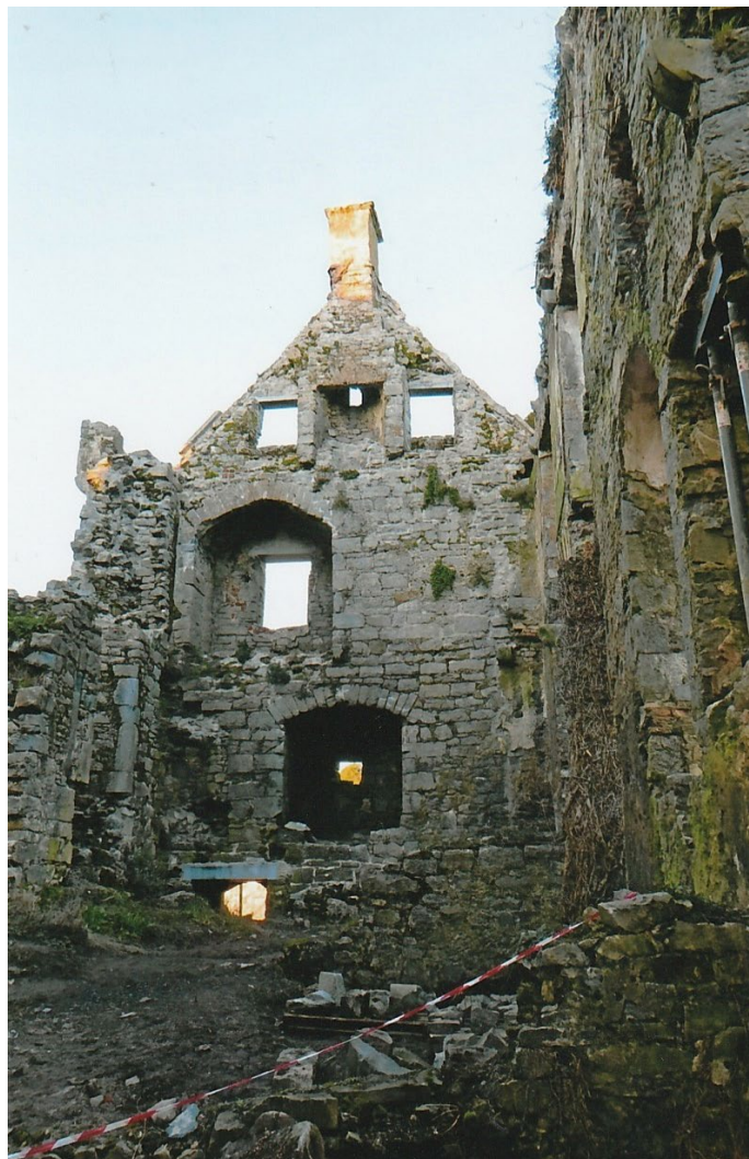
Fig. 105 Part of the Hall House Castle-cum-Tower House partly consolidated in 2022. Photograph: J. Higgins.
