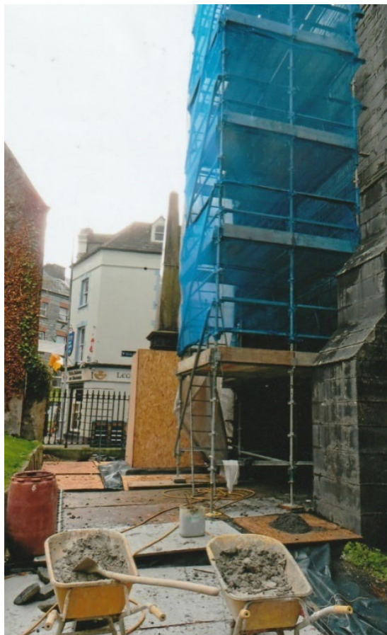
Fig. 1 The scaffolded area of the 16 th century southern extension to the south transept of St. Nicholas' Collegiate Church. The extension consists of the area to the left of the buttress shown in the photograph.
