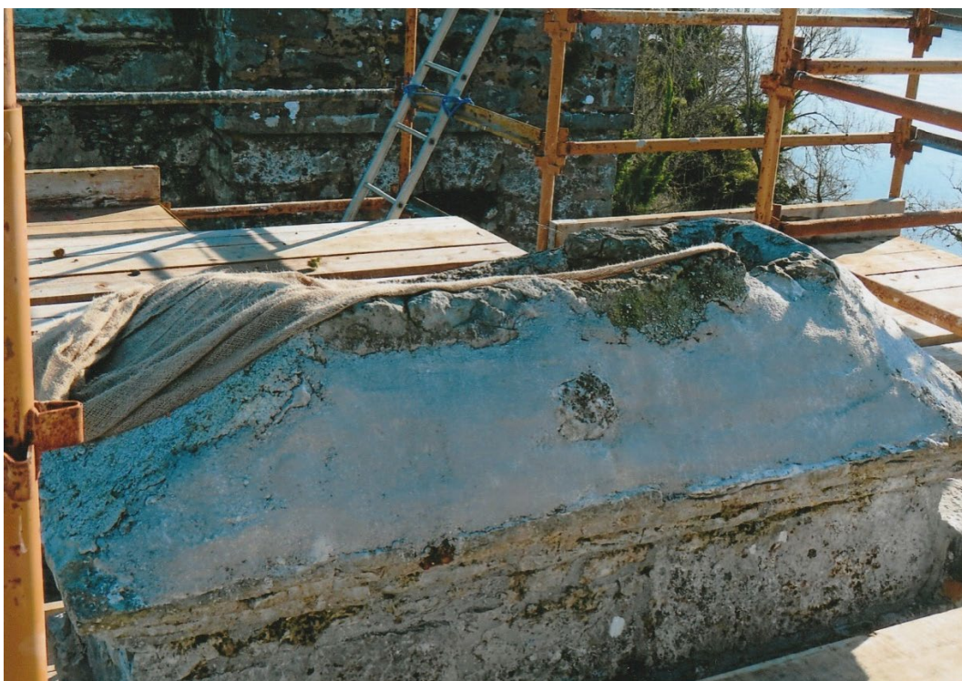
Fig. 77 Repairs to one of the Menlo Castle chimney stacks in 2023. Photograph: J. Higgins.
