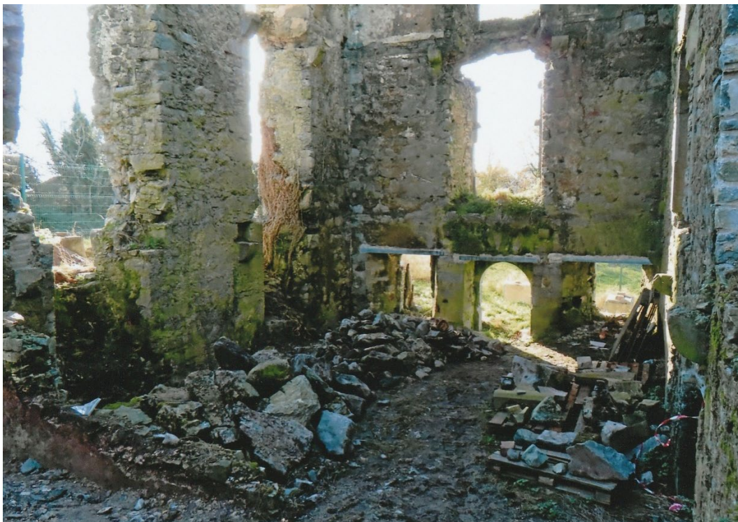
Fig. 76 The interior of the 17 th century block of Menlo. Fallen stone and rubble was sorted and architectural fragments were put on pallets in 2022 and 2023. Photograph: J. Higgins.
