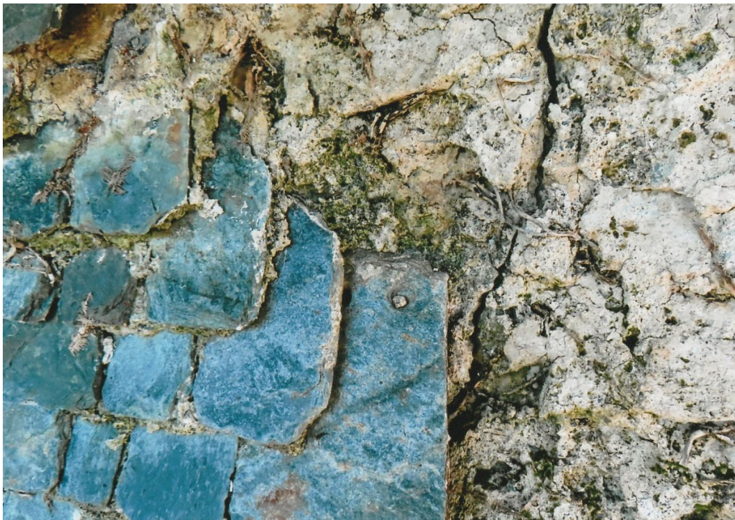
Fig. 90 Some of the surviving schist weather sheeting bedded in lime mortar some have nail holes but are reused. Note the remnants of ivy roots. Photograph: J. Higgins.
