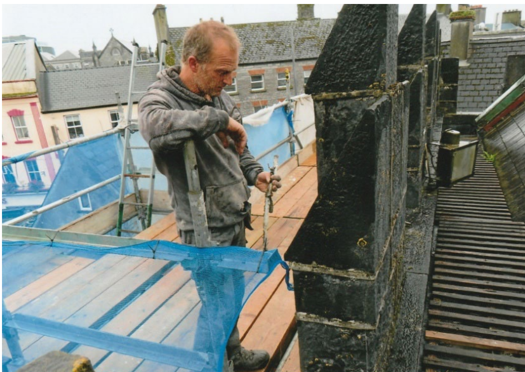
Fig. 32 Removing mastic “strip pointing” in some areas mortar pointing had been used over mastic and was failing. Photograph: J. Higgins.
