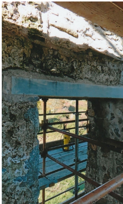
Fig. 74 A limestone lintel inserted over a window. The original lintels had rotted out but were circular logs of wood cut in half.
