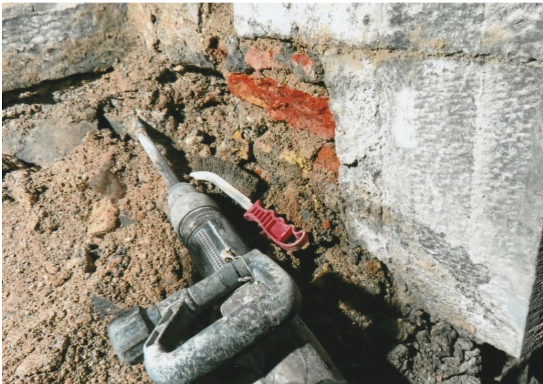
Fig. 14 The ingoing of the upper window part of the window is rebuilt. The block of ashlar and brick on the right are indications of repair or rebuilding. Note the post-medieval tooling on the stone. Photograph: J. Higgins.
