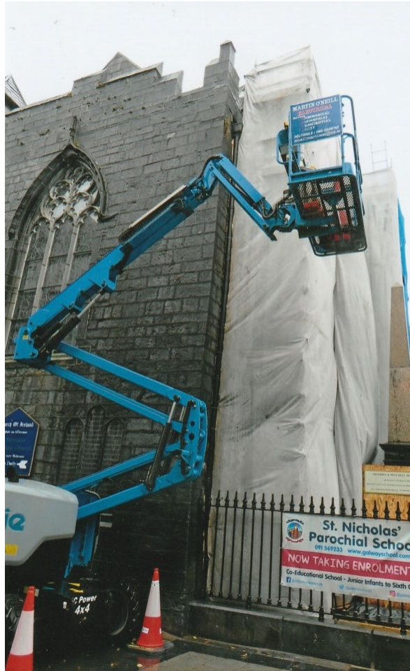
Fig. 11 Scaffolding on the exterior of the southern extension to the south transept of St. Nicholas' Collegiate Church. Photograph: J. Higgins.
