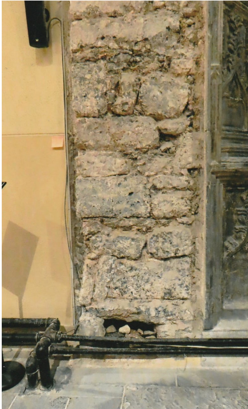
Fig. 64 The removal of some of the late mortar from a sample area of the lintelled ope to the left of the Flamboyant Canopied and Traceried Lynch tomb showed the presence of an ope with walling to the back of it.
