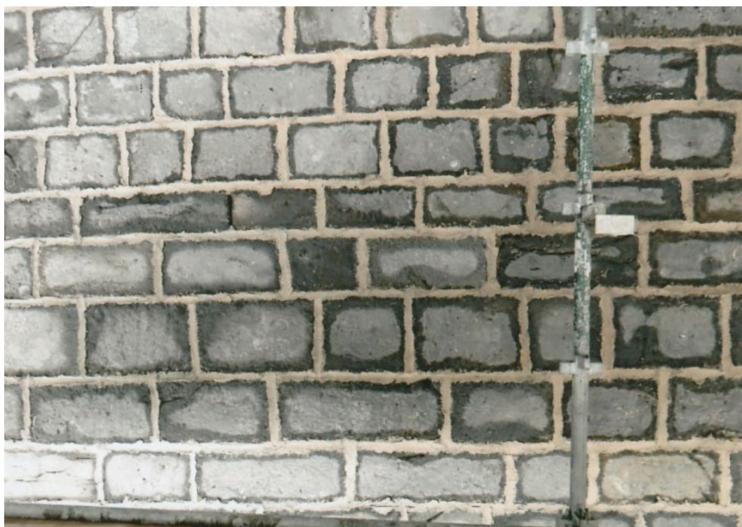
Fig. 29 Preliminary packing of joints with new lime mortar as part of the repointing process. Photograph: J. Higgins.
