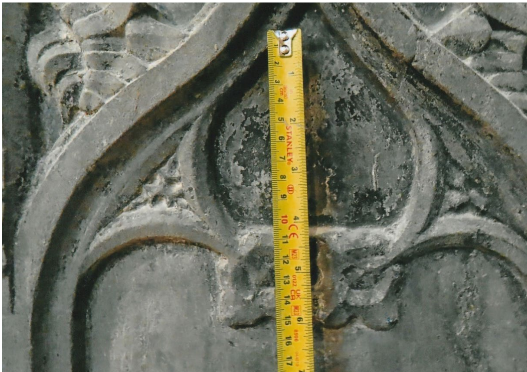
Fig. 63 Traces of eroded paint on the arcading of the Flamboyant Canopied and Traceried Lynch Tomb.
