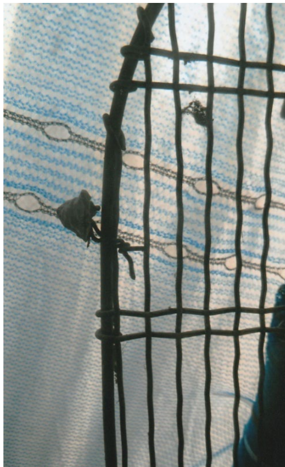
Fig. 49 The window grills were removed and now copper alloy ties and lead plugs were used to replace the old ones shown here. Photograph: J. Higgins.
