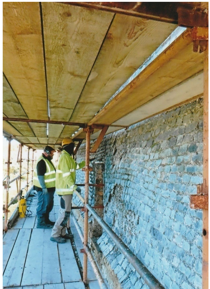
Fig. 88 The weather sheeting of schist (with some blue Bangor slate repturs extended over string courses on the river side façade of the castle and must have produced a glimmering shiny effect which contrasted with the white render of the lower façade. Photograph: J. Higgins
