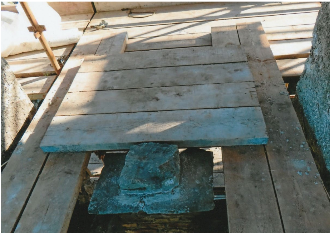
Fig. 79 Scaffolding and planking around decorative finials of brick and stone on the River front of Menlo Castle. The brick was Annaghdown – Clonboo brick and had previously been rendered in lime mortar and harling.
