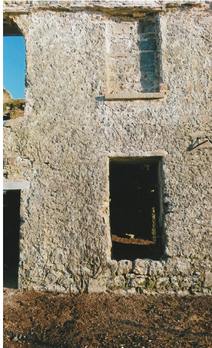
Fig. 96 Ground floor window with relieving arch above a lintel. Part of the lower walling of this frontage may be late medieval. The upper, blocked window is 18th – early 19th century. Photograph: J. Higgins.
