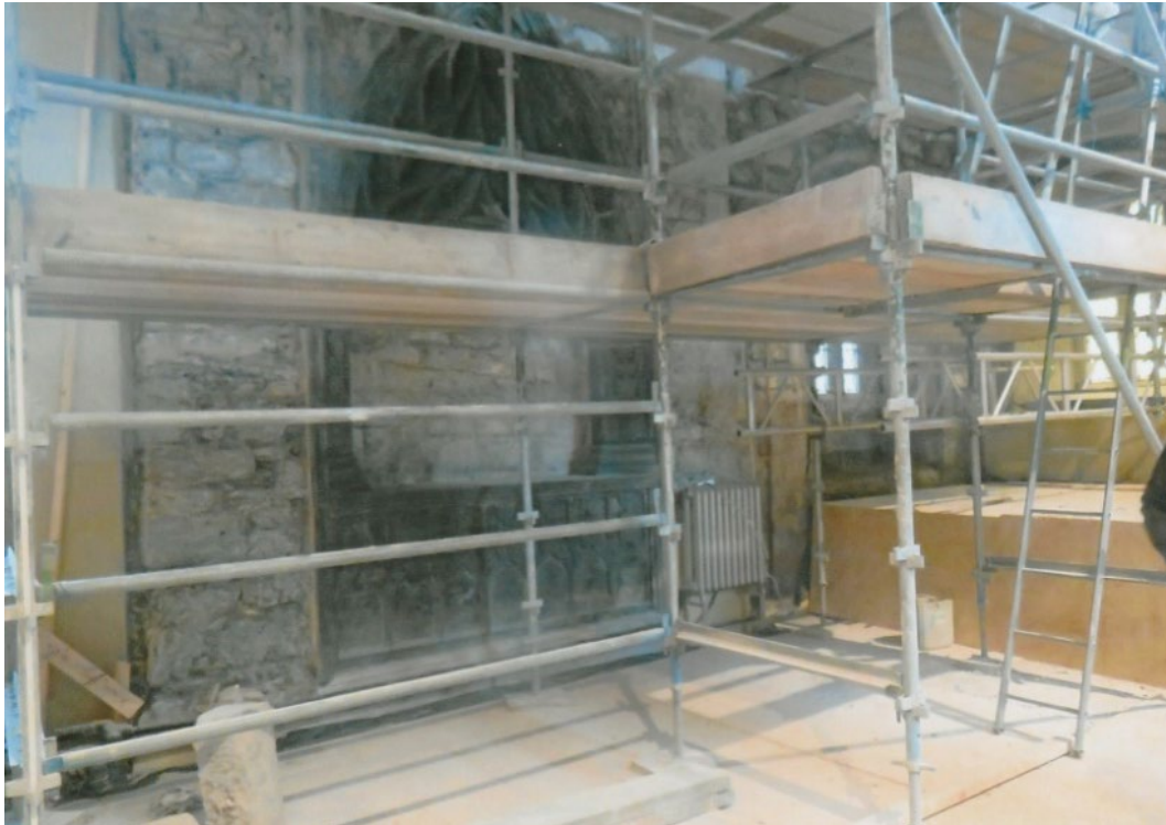
Fig. 48 The scaffolded area in the South Transept Extension. In the east wall the Flamboyant tomb projects from a rectangular area of walling (left). The Lynch Corner-tomb (right) has been boxed in with wood. The windows above the tomb and the area above and around the Flamboyant Lynch tomb were stripped of modern mortar which was trapping moisture. Photograph: J. Higgins.
