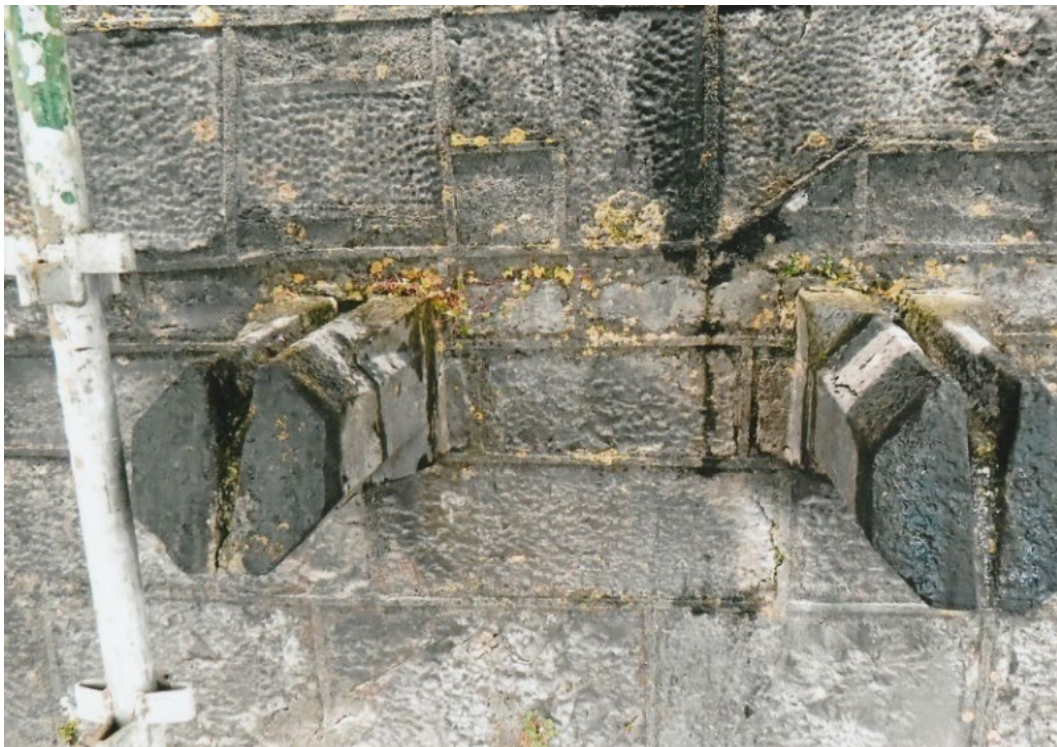
Fig. 35 The water spouts and stonework on the exterior of the south transept extension before the removal of the 1950's – 1960's raised pointing. Photograph: J. Higgins.
