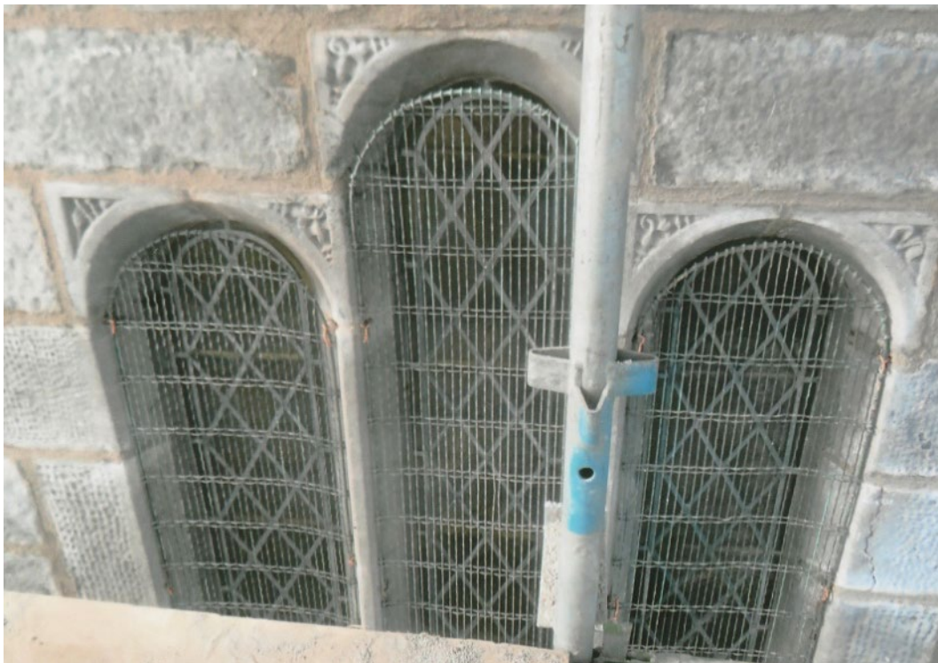
Fig. 47 The 1950's – 1960's grills repositioned on the windows. Photograph: J. Higgins.
