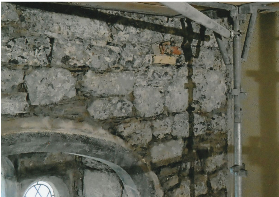
Fig. 56 Brick filled socket above the upper window in the South Transept Extension (upper right corner). Photograph: J. Higgins.
