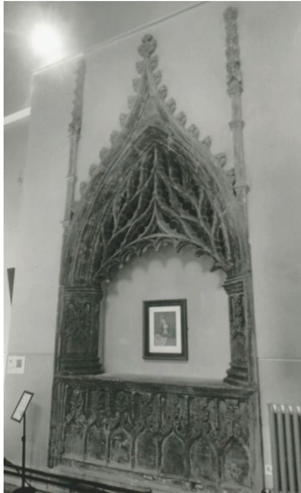
Fig. 40 The Flamboyant Canopied and Traceried Lynch Wall Tomb prior to commencement of works.
