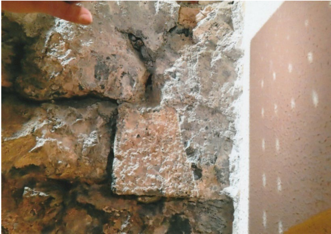
Fig. 34 The remains of the right hand corbel or bracket from which supported the gallery from Lynch's stair turret across the South end of the South Transept Extension.
