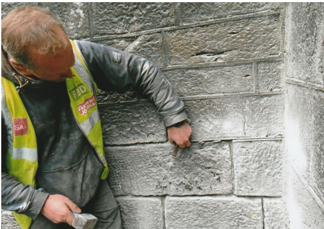
Fig. 27 Cleaning the joints after the ribbon-pointing was removed. Photograph: J. Higgins.
