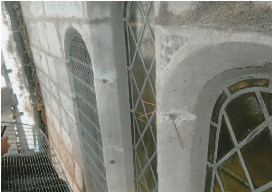
Fig. 46 New copper ties set in lead to hold the window grills of the exterior windows of the South Transept Extension. Photograph: J. Higgins
