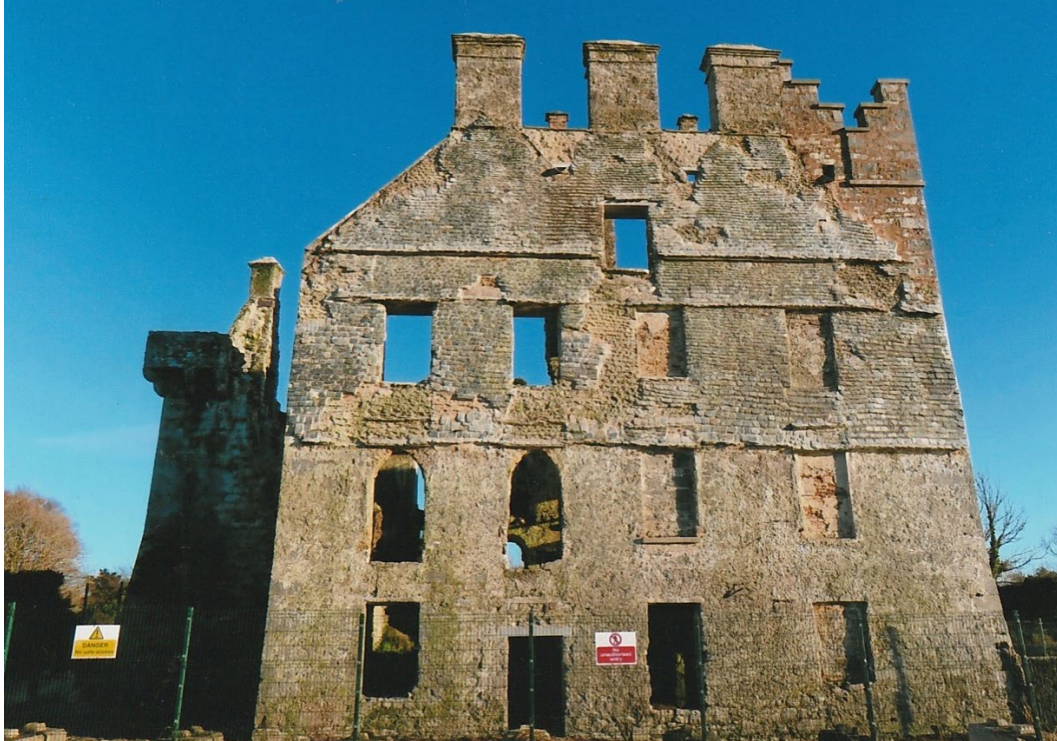
Fig. 94 The exterior face of walling consolidated in 2023. Photograph: J. Higgins.
