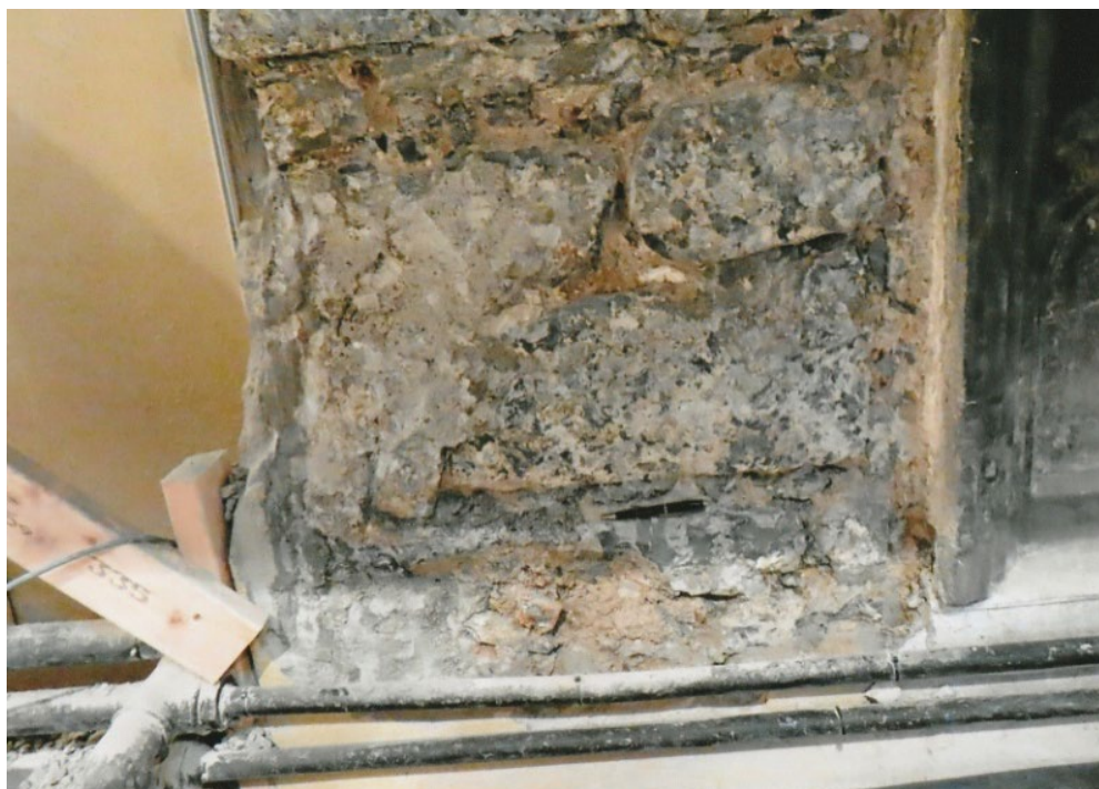
Fig. 4 Part of the rectangular surround to the flamboyant canopied and traceried wall tomb or wall frame. This incorporates reused stone of 12-14th century date as well as 15th and 16th century material. The stone with the pen on it projects by about 6cms from the wall face and has two wedge-like stones similar to a relieving arch on top of it. This is a broken lintel, a crude fill below it. It is possible that there was an entrance to a vault here. Photograph: J. Higgins.
