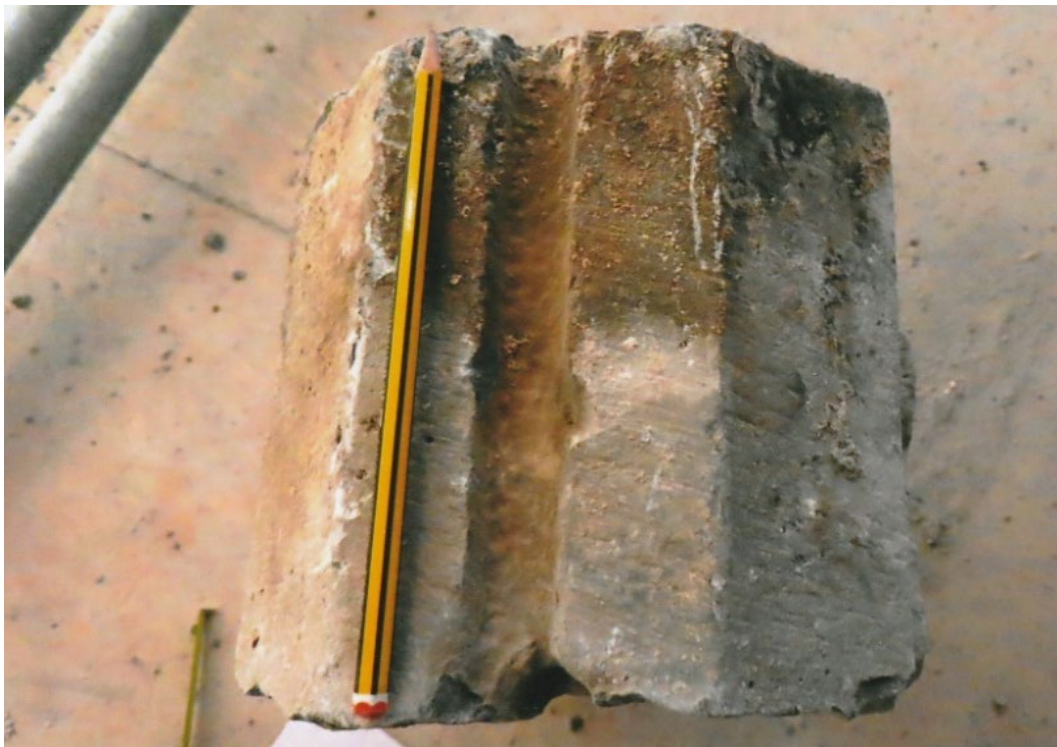
Fig. 16 Detail of the mullion showing the thin tooling on the general surface and pecked within the glazing groove. Photograph: J. Higgins.
