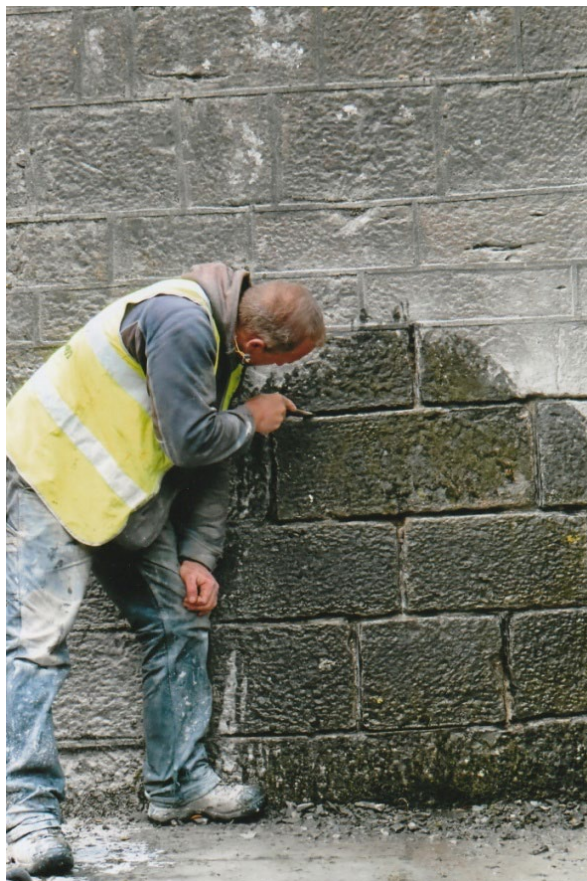
Fig. 3 Laurik Mathieu, Conservation Stone Mason raking out joints on the exterior of the south transept extension. The raised ribbon pointing was applied during works carried out between 1958 and 1962. Old photographs taken before that date show flush pointing with eroded lime mortar pointing. The raised ribbon pointing has trapped moisture in the core of the wall. Photograph: J. Higgins.
