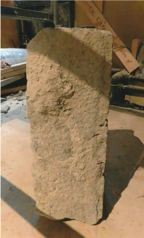
Fig. 21 A&B Two sides of an ashlar block with a thin coat of 1950's – 1960's cementitious shuttering from the ground floor window of the south transept extension. The ashlar block is probably of the 14th to 15th centuries. Photographs: J. Higgins.
