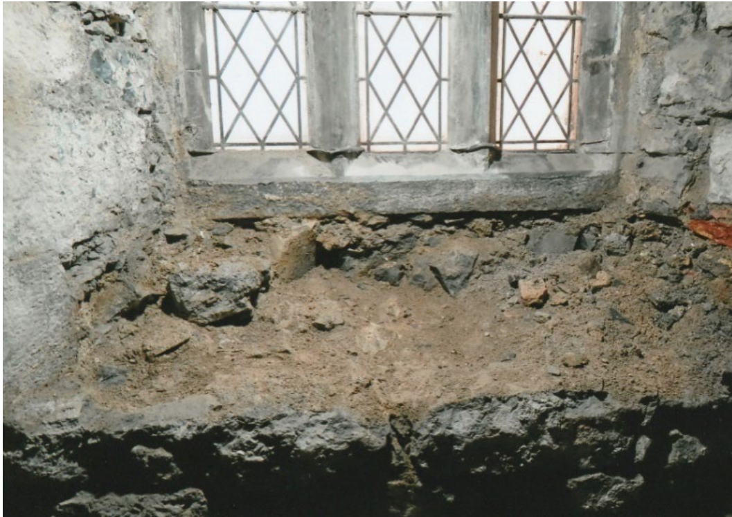
Fig. 13 The inclined base of the ingoing of the upper window of the south transept extension after the removal of the 1958-62 concrete capping. Note the red brick in the right side of the ingoing. Photograph: J. Higgins.
