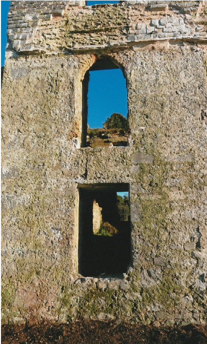
Fig. 95 Georgianised Gothic Revival window and below enlarged window with possible earlier features. Photograph: J. Higgins.
