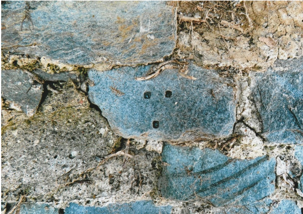
Fig. 89 Not a plug socket! Just old holes in some of the schist weather slating at Menlo Castle. Photograph: J. Higgins.
