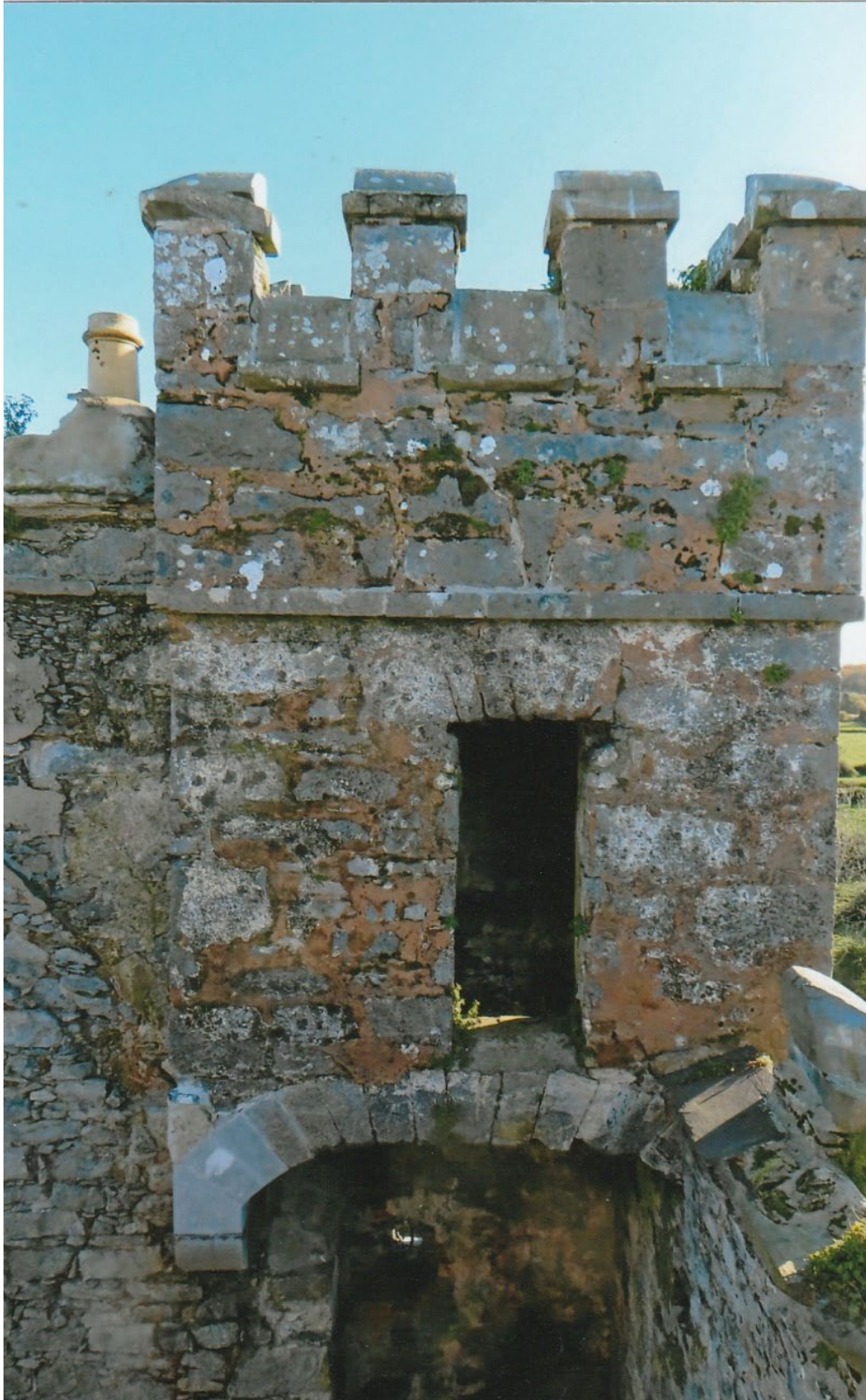
Fig 80 The 19 th century crenellated turret or Belvedere at Menlo Castle. This was supported on an arch and projected over 18th century fabric. The arch needed re-supporting and two new voussoirs, a o shew-back and a very large curved-fronted corbel were inserted in 2022 by Galway Stone Design to replace lost features.
