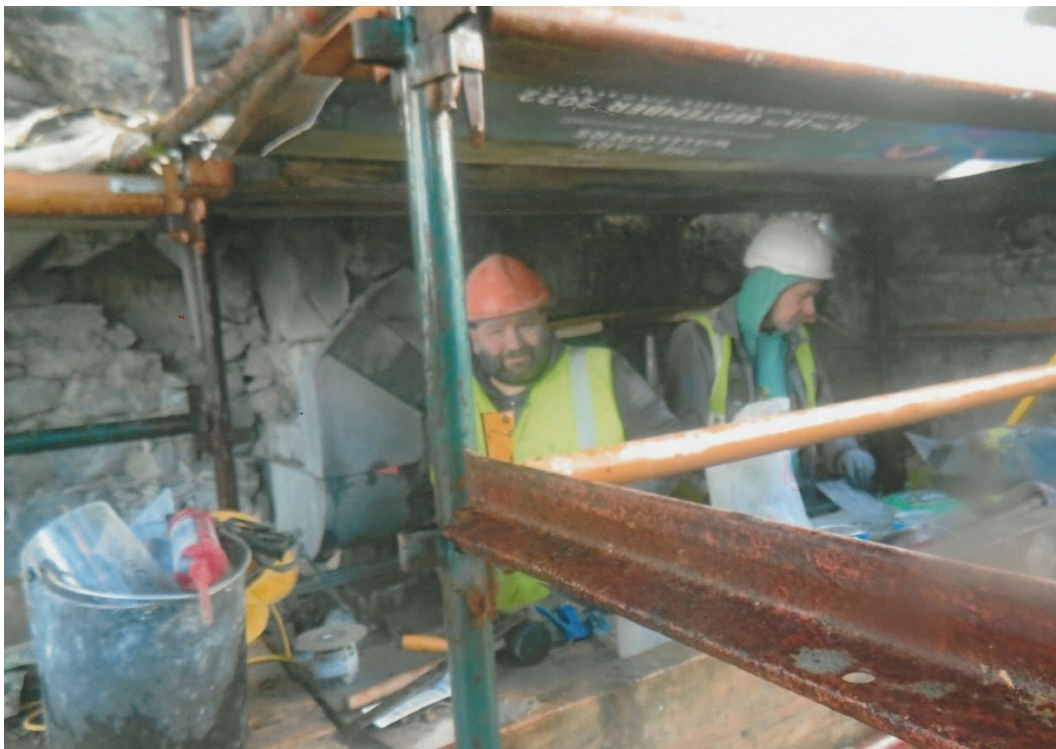
Fig. 81 Sebastian and Kris of Galway Stone Design inserting the voussoirs and corbel to support the Turret in 2022.
