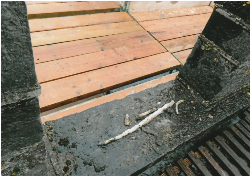
Fig. 31 In the last few decades the crenellations had been “pointed” with mastic and cementations and non-cementations raised bands. These inappropriate materials have been removed. Note the post-medieval string course on which the crenellations had been set. Photograph: J. Higgins.
