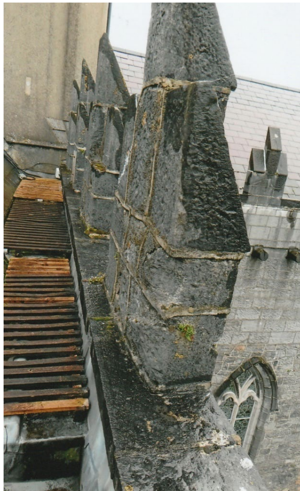
Fig. 37 The wooden duck-walk behind the parapet covers a metal drainage trough with feeds into the hopper at the top of the cast iron down pipes.
