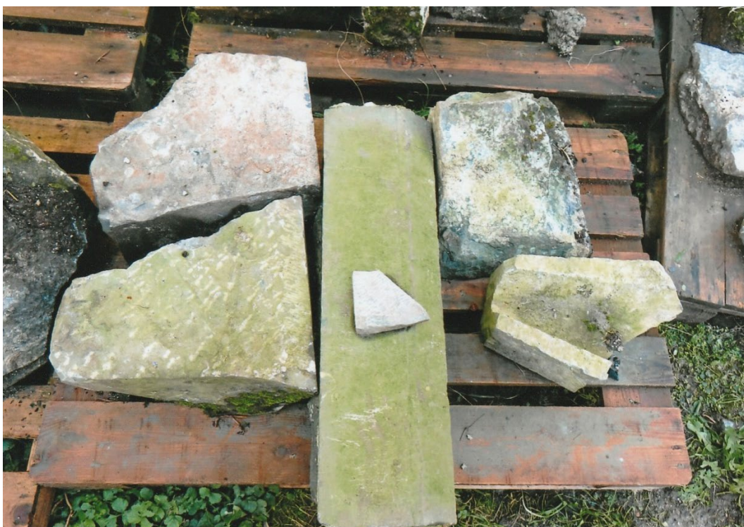
Fig. 84 Window, door and water spout fragments on pallets in 2023. The tapering water spout comes from a broken water spout on the 17 th century frontage and will be put back in position. The window fragment in the middle was found in 2022. A full catalogue of architectural fragments is in preparation.
