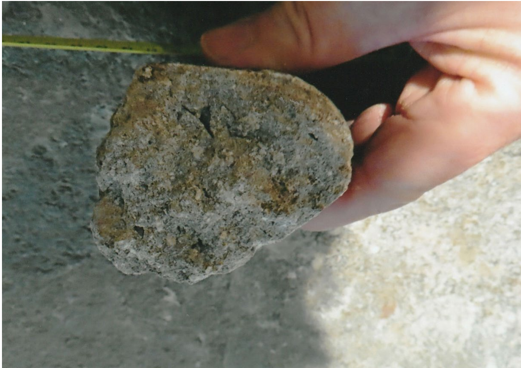
Fig. 65 A piece of moulded plaster moulding found in the recess below the Lynch Canopied and Traceried Wall Tomb.
