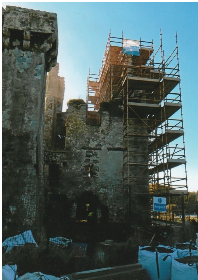
Fig. 92 Scaffolding at Menlo Castle in October 2023.
