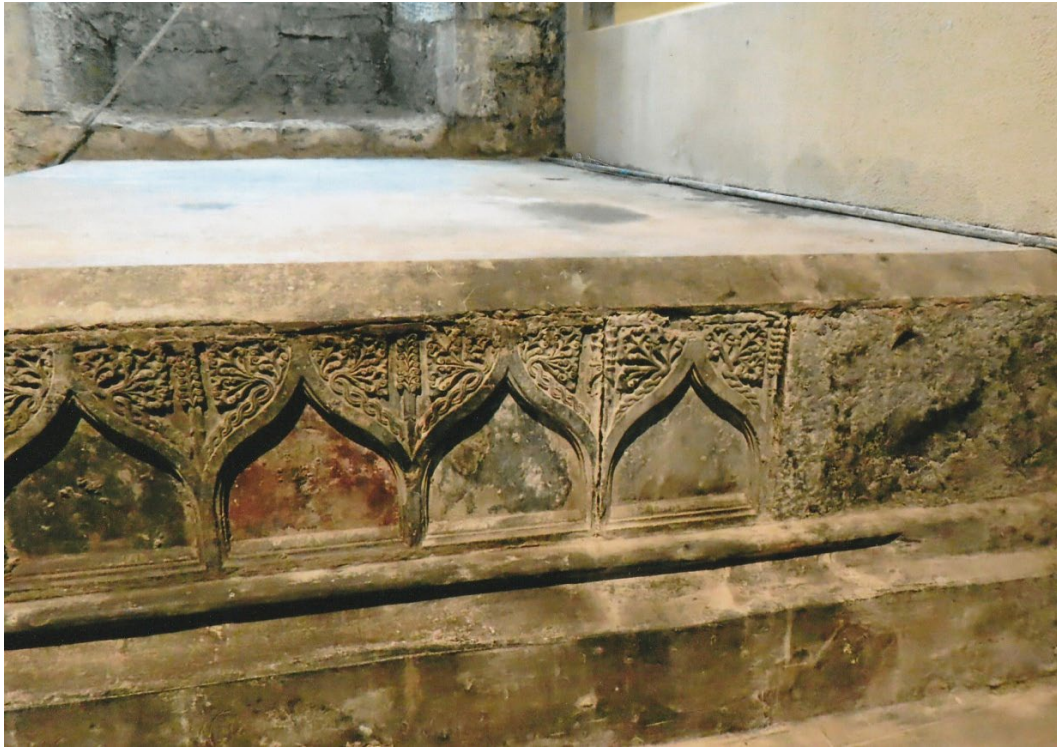
Fig. 60 The Lynch corner tomb in the S. Transept with a blank panel on the right. The concrete capping predates the 1950-1960's works and seems to have been added in the late 19th century.
