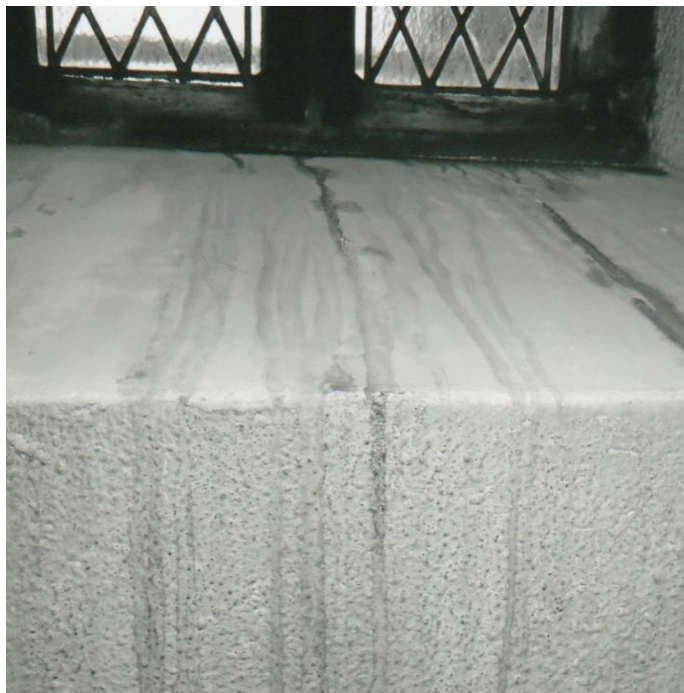
Fig. 69 Water flowing from a window sill in the South Transept of St. Nicholas' Collegiate Church October 2023. The window embrasures were filed to the base of the interior of the sills prior to the 1950's – 1960's re-rendering of the interior of the church. Photograph: J. Higgins.
