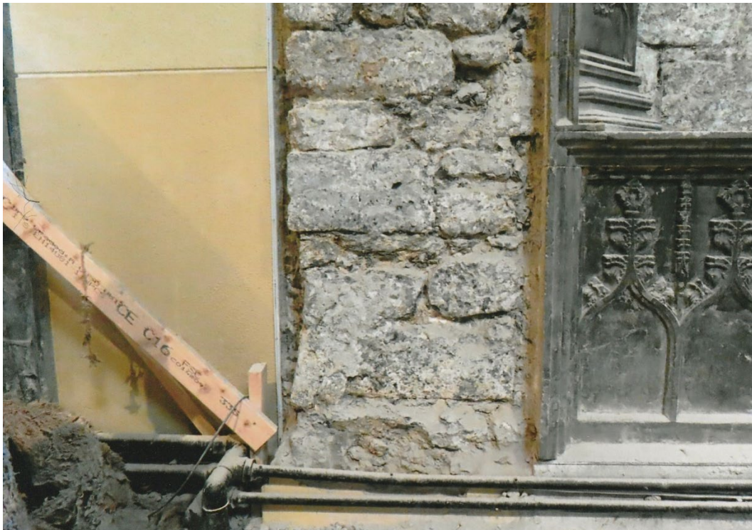
Fig. 55 The blocked ope, truncated lintel and relieving arch to an opening to the left of the base of the Lynch Tomb.
