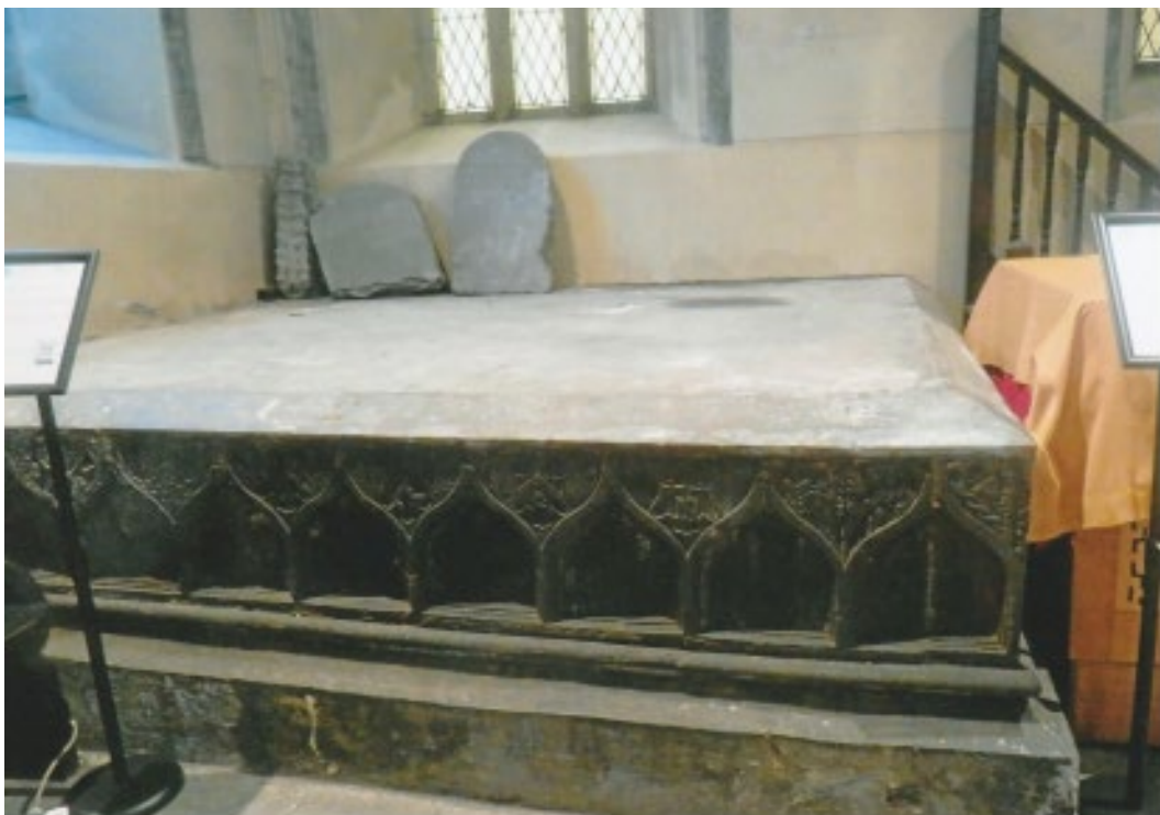
Fig. 41 The Lynch Corner-tomb in the South Transept Extension prior to commencement of Conservation works. Photograph: J. Higgins.
