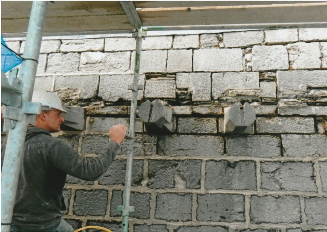
Fig. 36 The removal of the 1950's – 1960's pointing has shown several phases in the water management features above the string course on top of the spouts the entire parapet was rebuilt.
