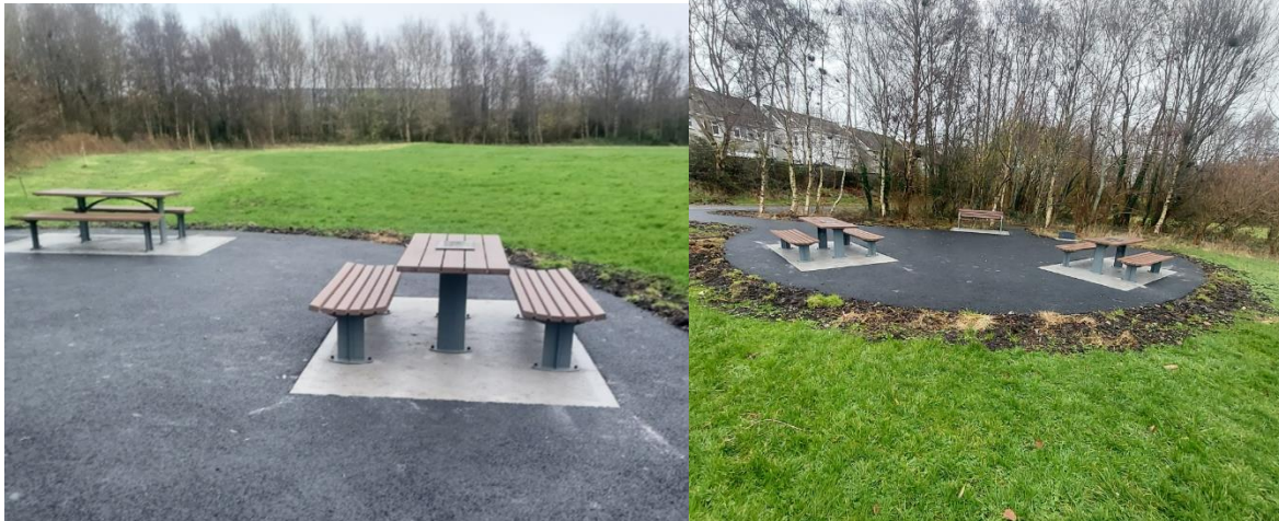
New picnic area with wheelchair accessible benches. Native species planting due in springtime.
