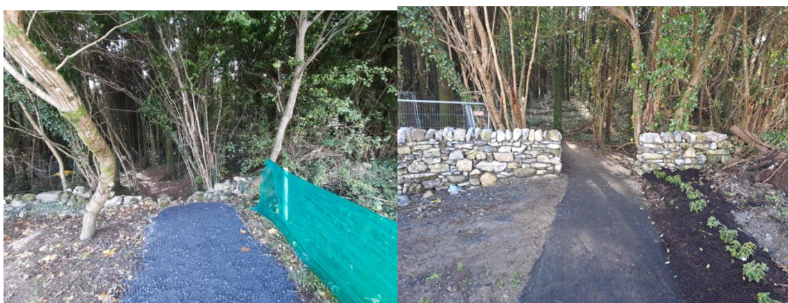
Before & After photos of access point at Fionnuisce and Merlin Woods
