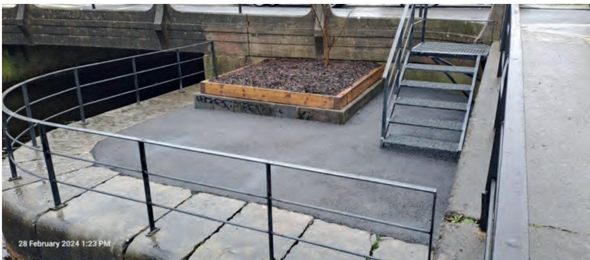
Resurfacing of recreational areas by the Eglinton Canal
