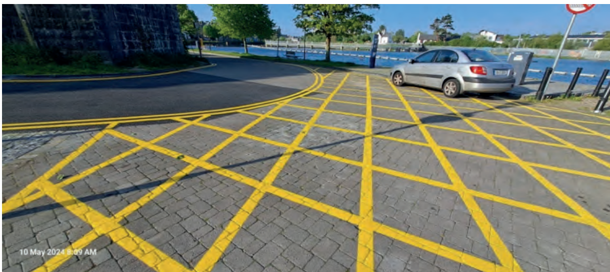
Steamers Quay paving after resurfacing and renewal of road marking works
